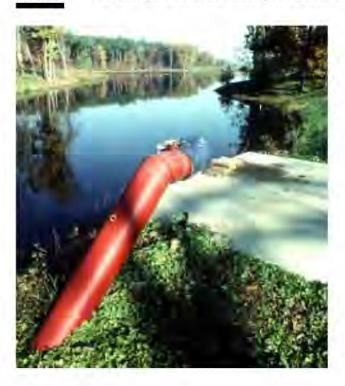
Figure 6 Details of a dry hydrant installation
