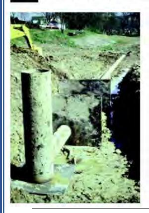
Figure 23 Drop-inlet pipe spillways
